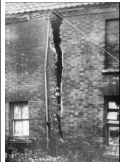
Fig 14. (left) The crack width adjacent to the window frame is about 60mm. Clearly the building is no longer watertight and the thermal insulation is being compromised. In time the construction materials will degrade
