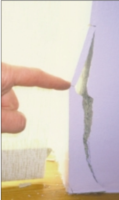
Fig 4. (above) Crack caused by shear
