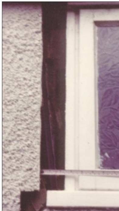
Fig 14. (left) The crack width adjacent to the window frame is about 60mm. Clearly the building is no longer watertight and the thermal insulation is being compromised. In time the construction materials will degrade
