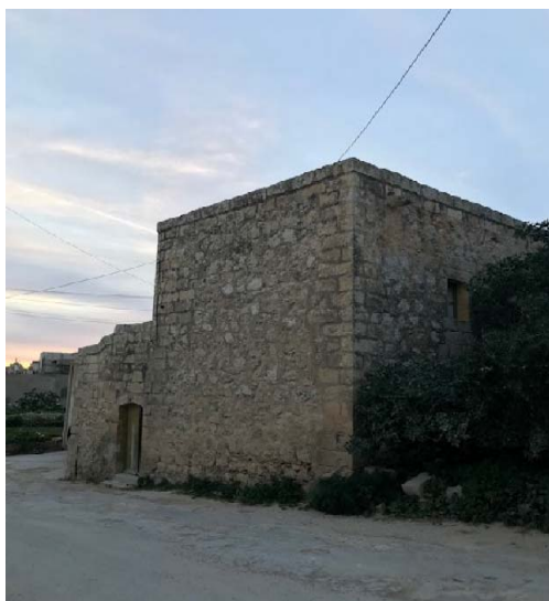
Figure 4: Construction in Gozo, note rubble infill walling with ashlar at the corners, together with the top string ashlar course. (SOURCE: Author)
