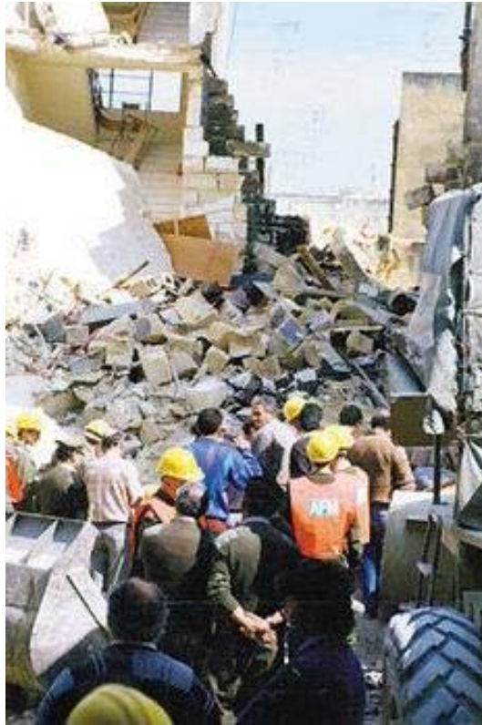
Figure 11: The devastation that resulted following the arson “chemical” explosion that went wrong, and which brought down a block of apartments and shops (Paola 1992) [49].
