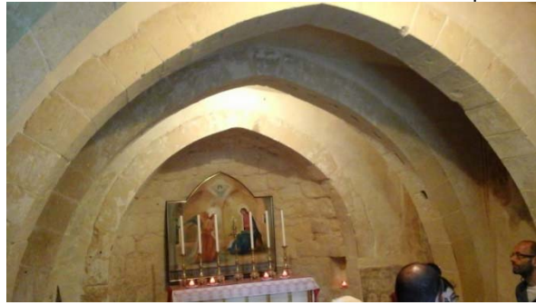
Figure 6: Chapel of Hal-Millieri in masonry construction Mqabba, consecrated 1480: 4.5m width, depth 7.5m on a 3.6m height – stone slabs spanning 1.525m onto masonry ashlar pointed arches, note rubble infill walling panels (SOURCE: Author).
